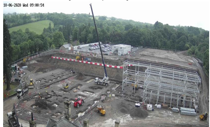
Overlooking the site from Hydro Building – Steelwork installation
